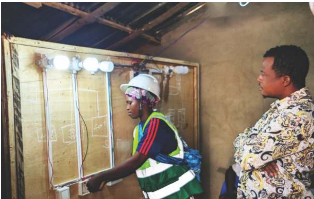
Huzaifa Bachandi, one of 3 girls enrolled for the electrical installation and maintaining livelihood skills training in Chereponi under the SURE Project
